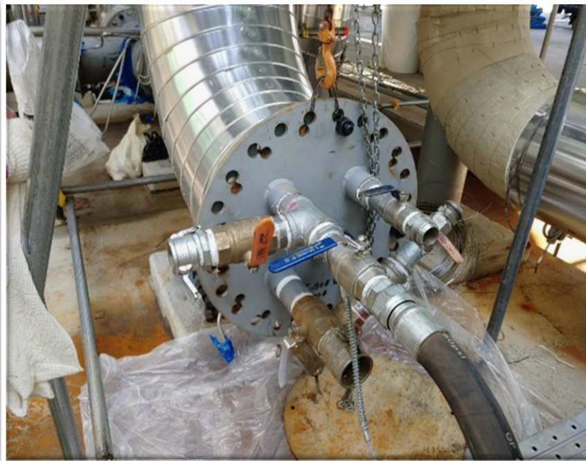
Launcher Trap (Blind)
