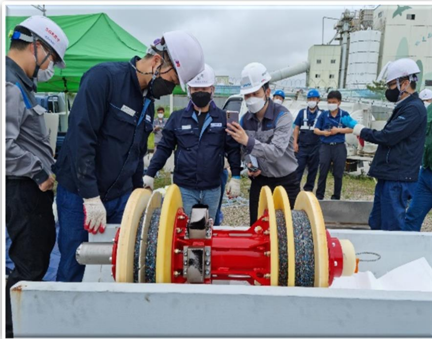
Disk Pig (Gauge) Inspection
