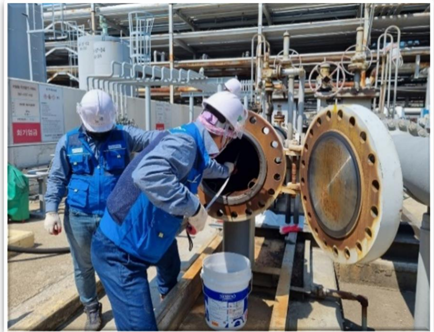
Disk Pig (Gauge) 장착
