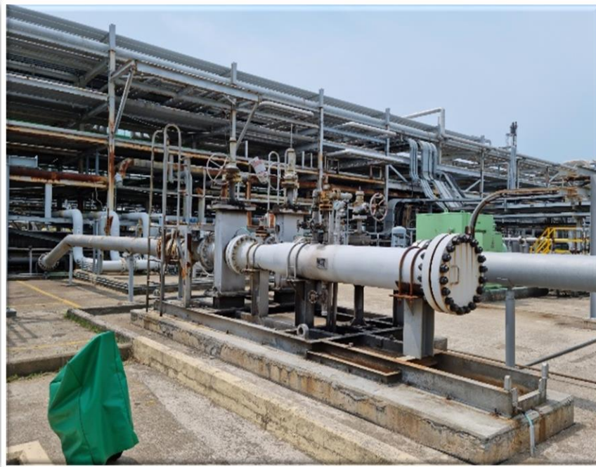
Intelligent Pigging Launcher
