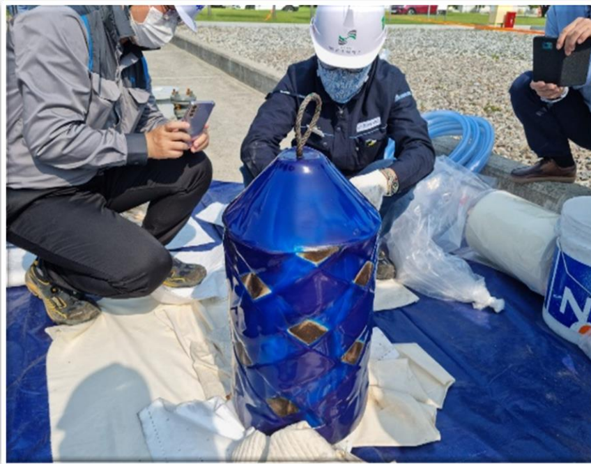
Foam Pig Inspection
