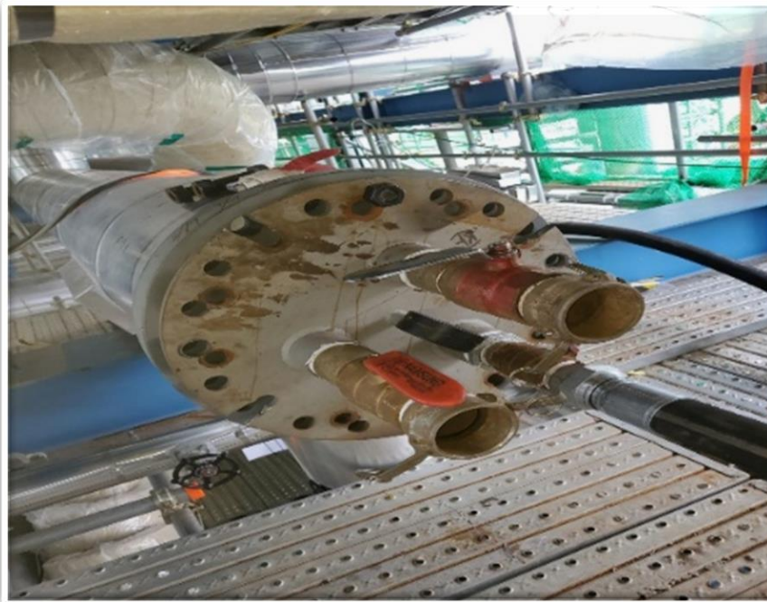
Launcher Trap (Blind)
