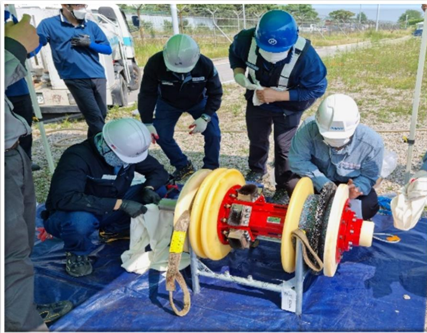
Disk Pig (Brush) Inspection
