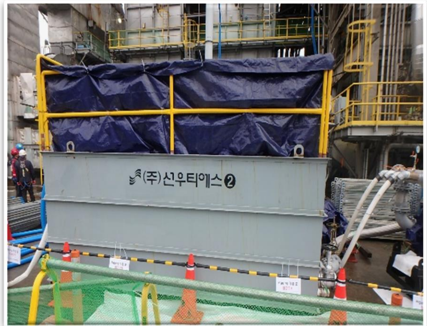
Decoking Water Tank
