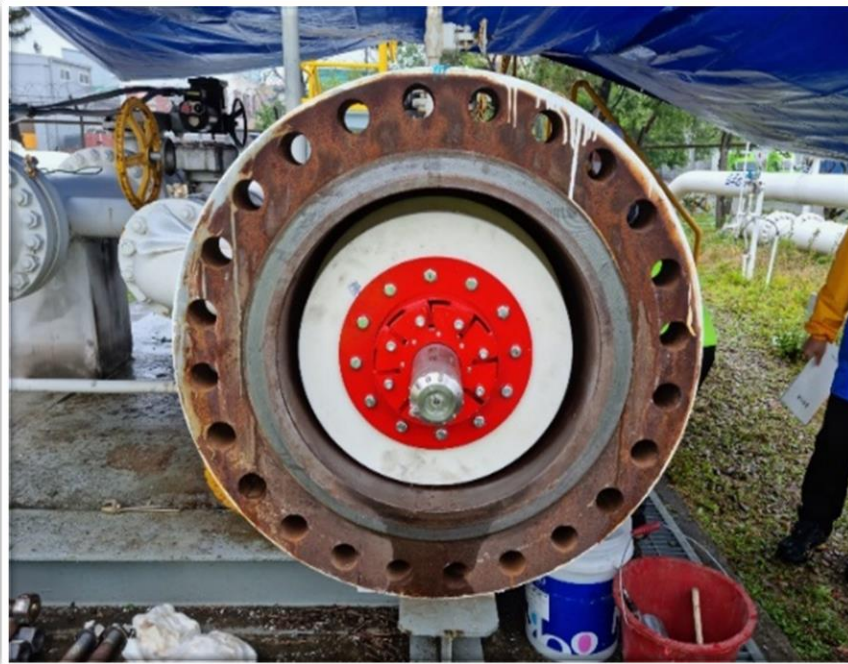
Disk Pig (Gauge) 장착
