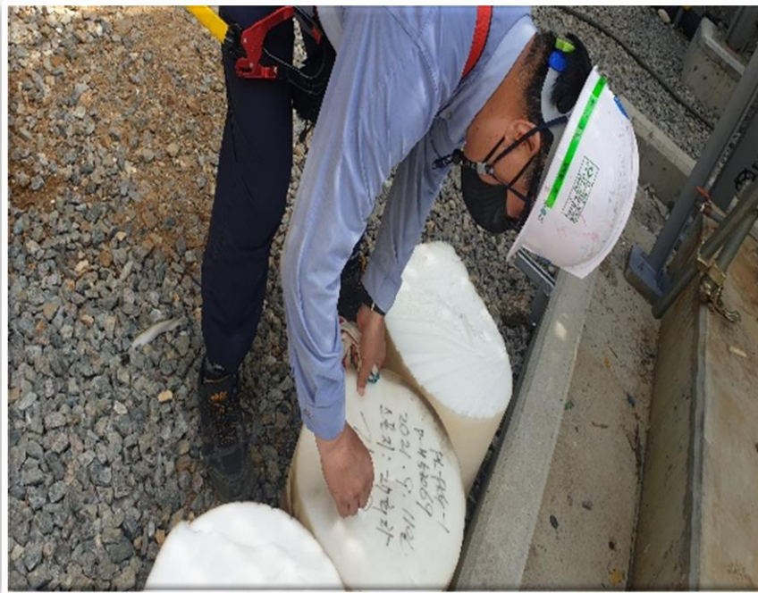
Sponge Pig Inspection
